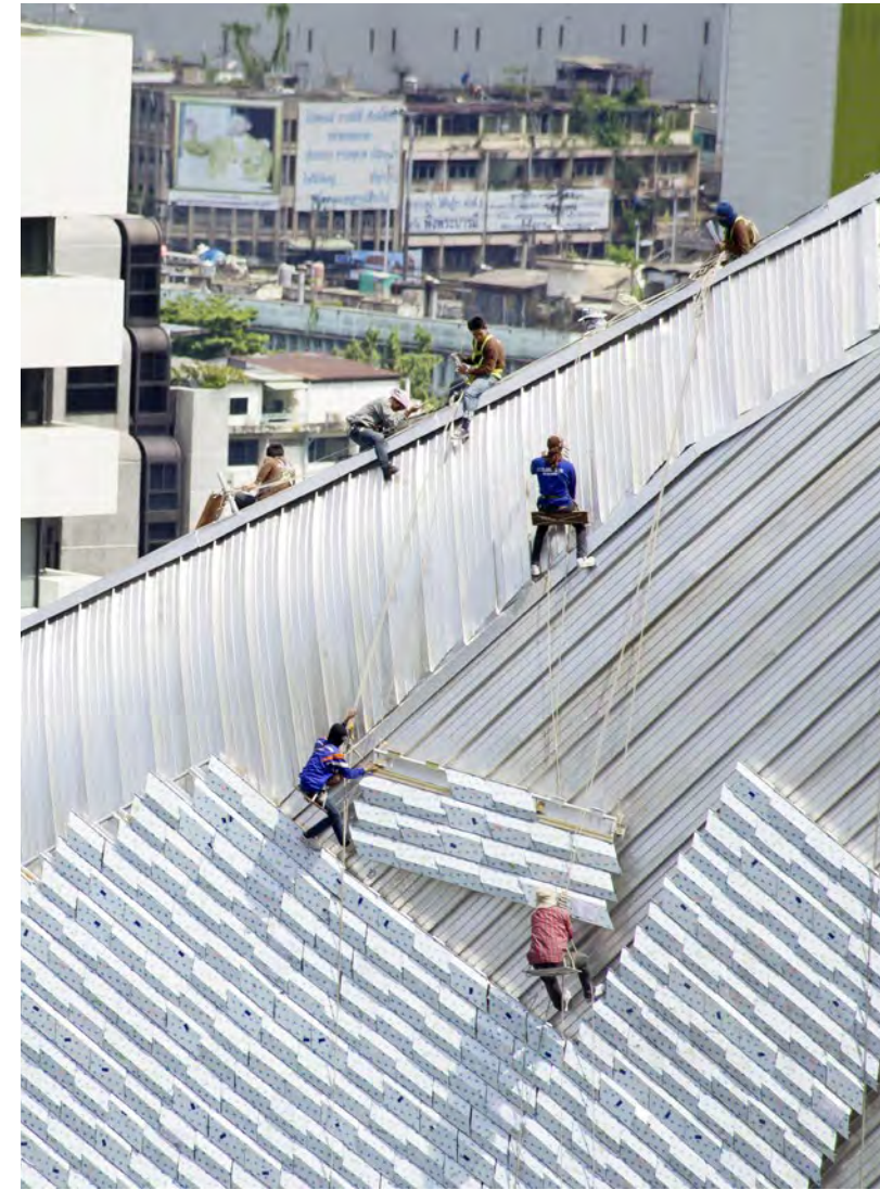
The tiles for the façade were clipped on to panels off-site.
